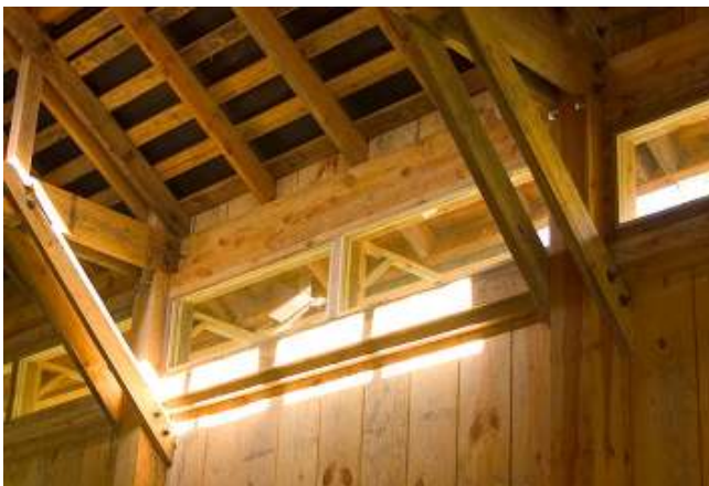
Locomotive Barn Inside
